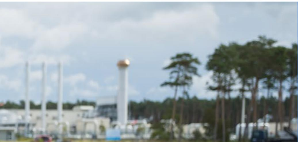
The station comprises two sections: the “offshore section” for the incoming Baltic Sea pipeline and an “onshore section” for the two downstream pipelines OPAL and NEL. The onshore section is subdivided into a “180 bar” and a “105 bar” section. The “180 bar” section has filters, pre-heaters and control valves, while the “105 bar” section features mainly measuring and control systems.
